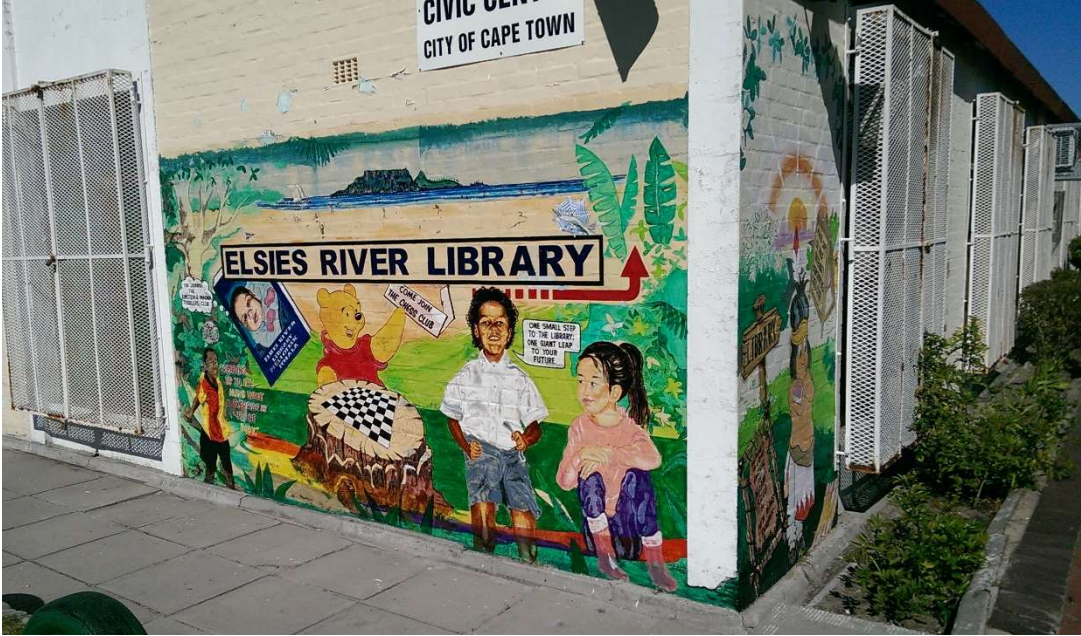
Figure 8 Elsie's River Library exterior
