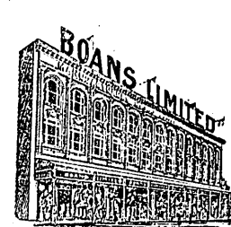
Wellington Street, Frontage
